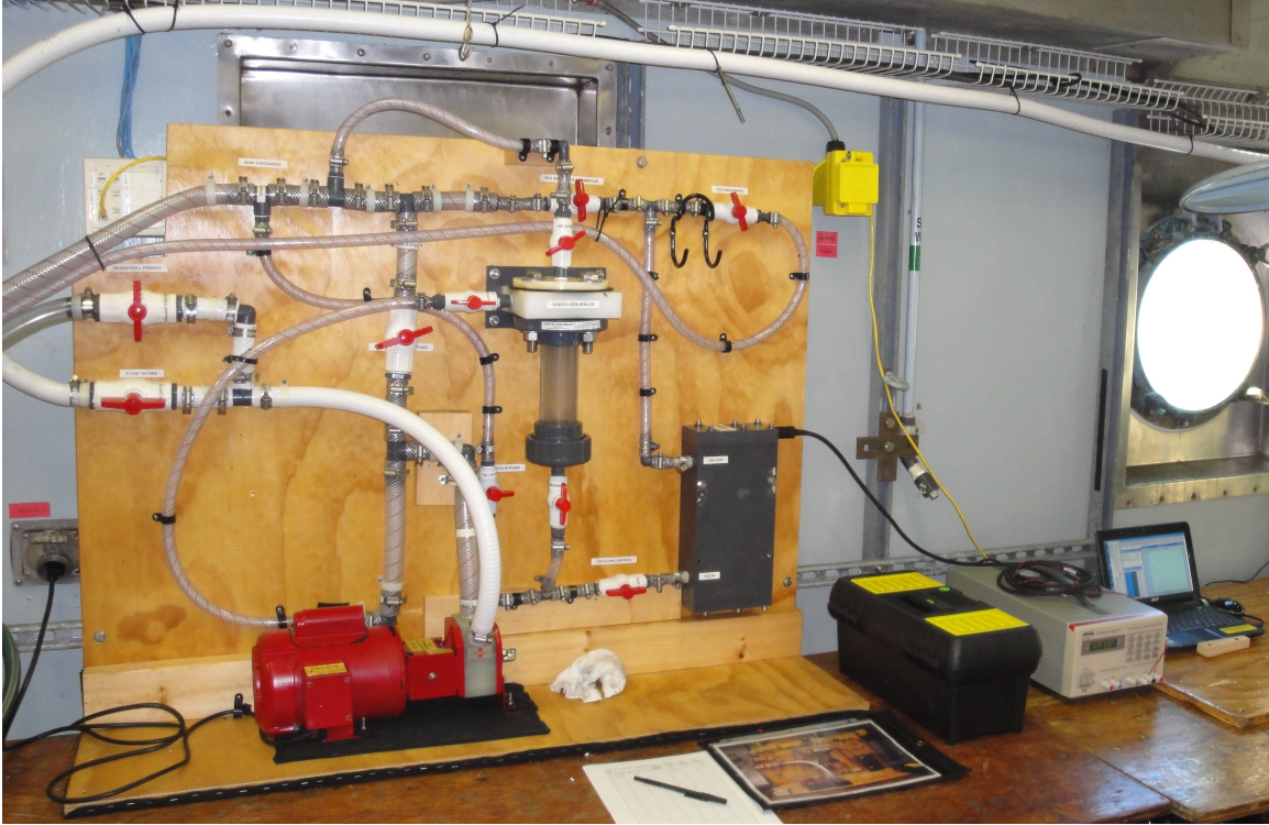
Figure 11.3: The interior sea snake plumbing, showing valve positions during normal operation.
