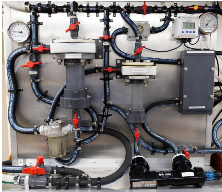
Figure K2: Shipboard system of the salinity snake, showing intake strainer, cascading vortex de-bubbler system, ultraviolet sterilizer, Seabird 45 thermosalinograph, flow meter and intake and discharge gauges.
